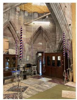
This photo shows a temporary rope guide installed above the second rope (in front of the clock) enabling the rope to be pulled away from the third rope (the rightmost rope shown). The third rope can also just be seen to have been pulled away from the fourth by movement of its guide on the arch.
